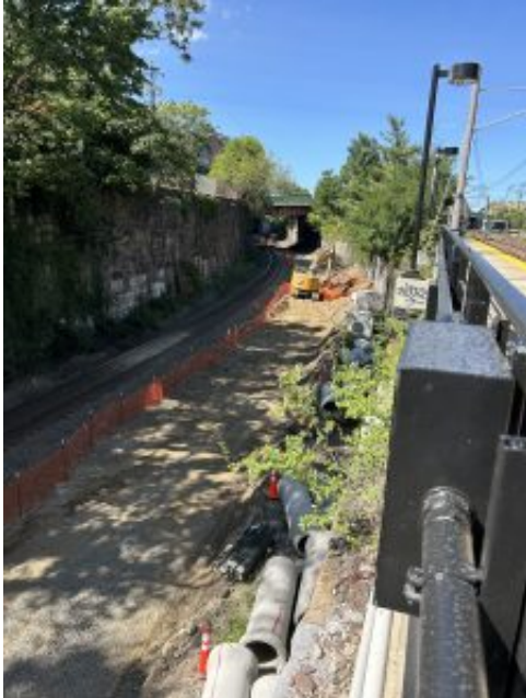
Track lowering work seen from the Light Rail Station
