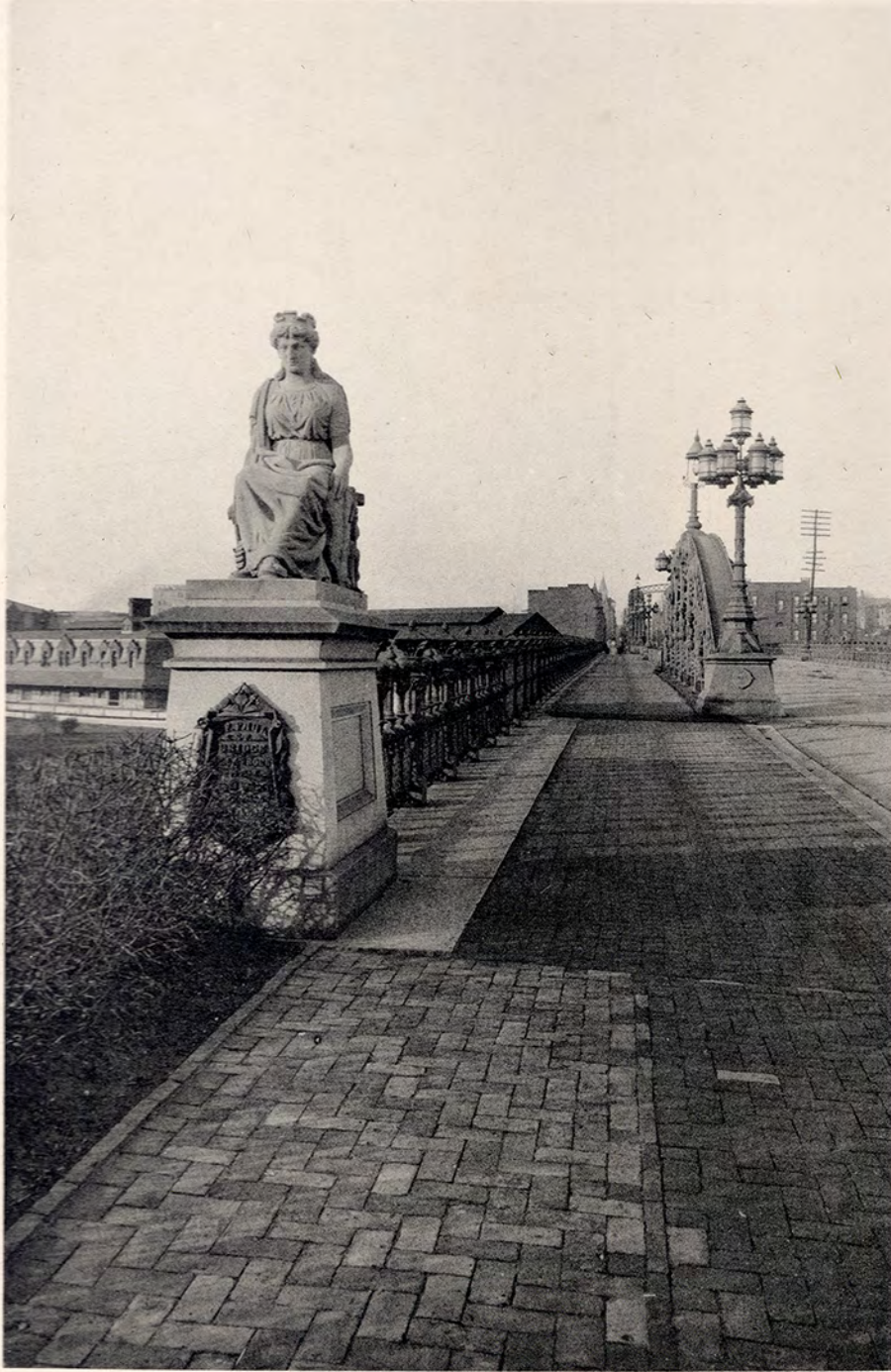
ST. PAUL STREET BRIDGE.
