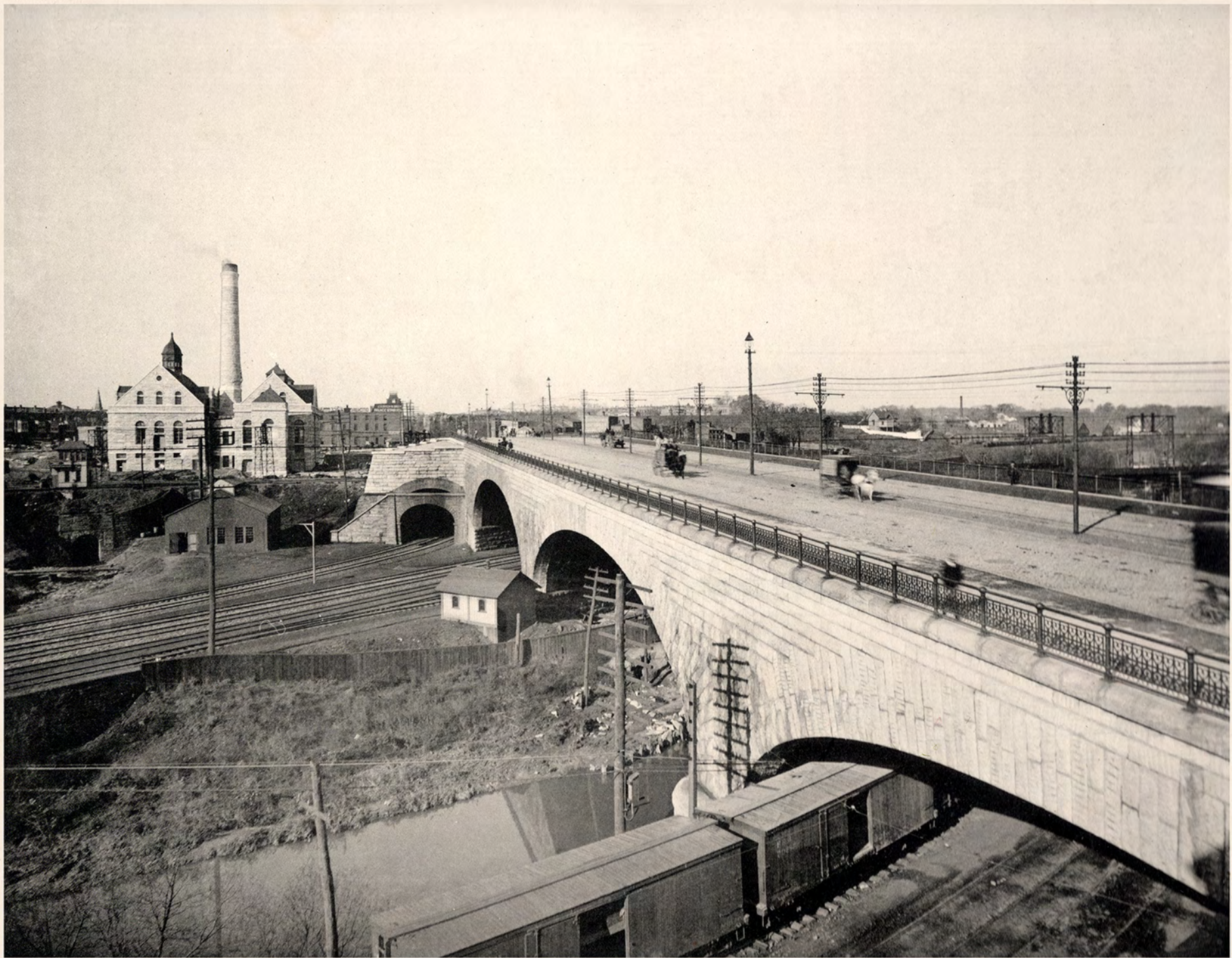
NORTH AVENUE BRIDGE.
