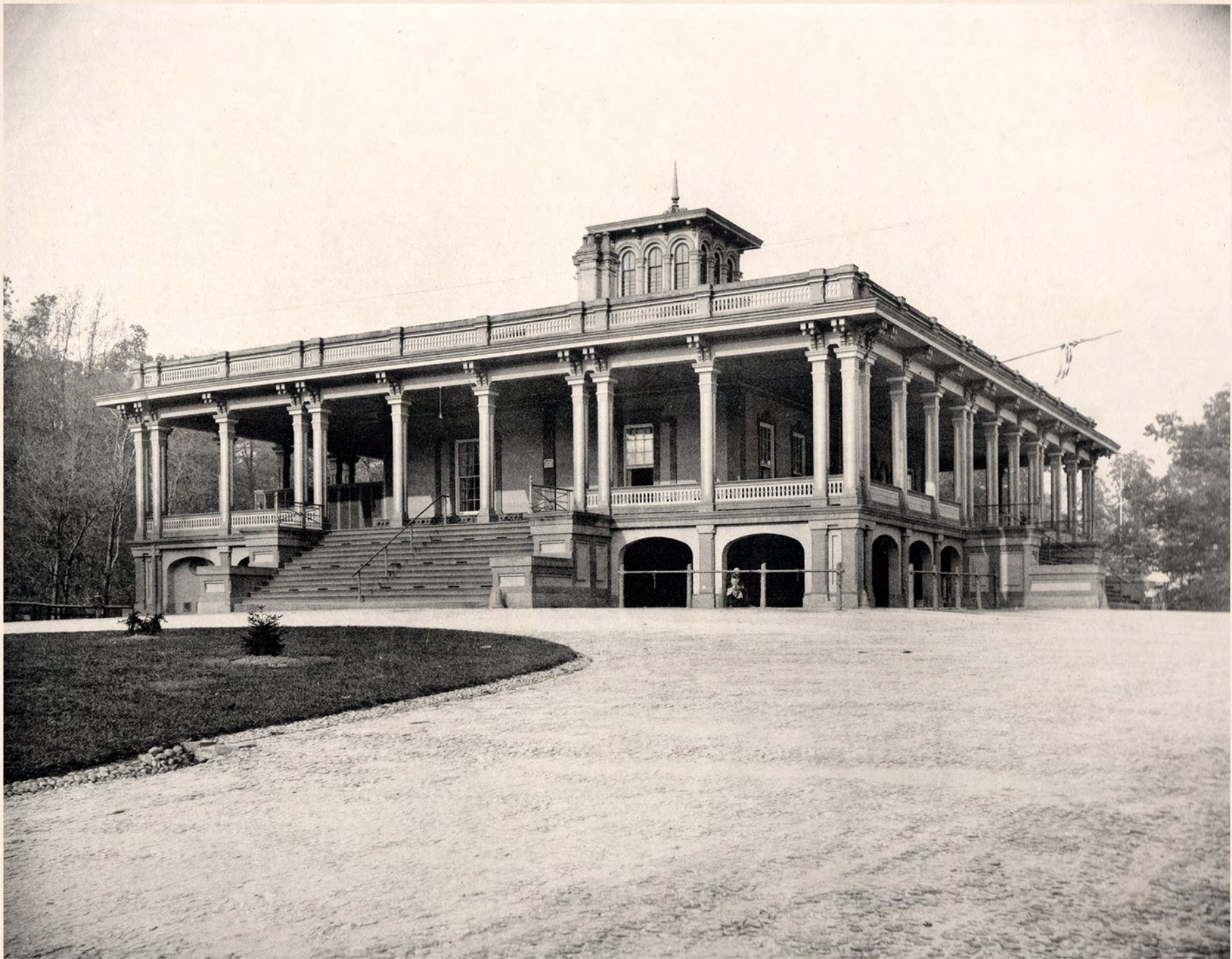
MANSION HOUSE - DRUID HILL PARK.
