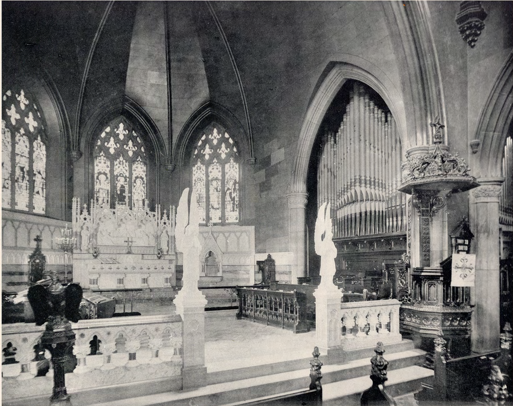
INTERIOR OF GRACE EPISCOPAL CHURCH.
