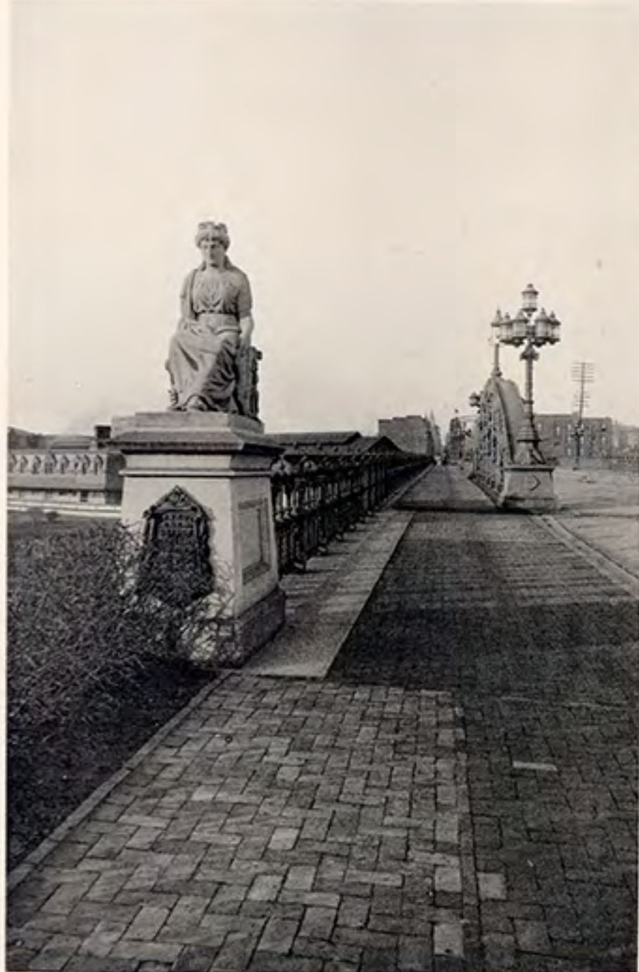
ST. PAUL STREET BRIDGE.
